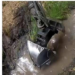
Small ditch building
