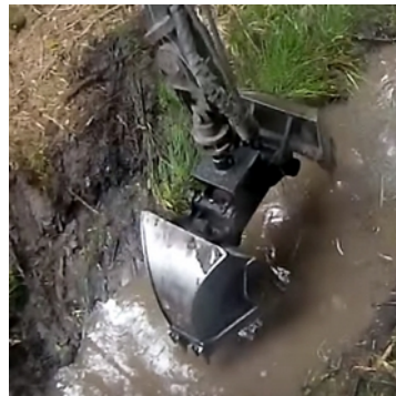
Digging and cleaning of ditches
